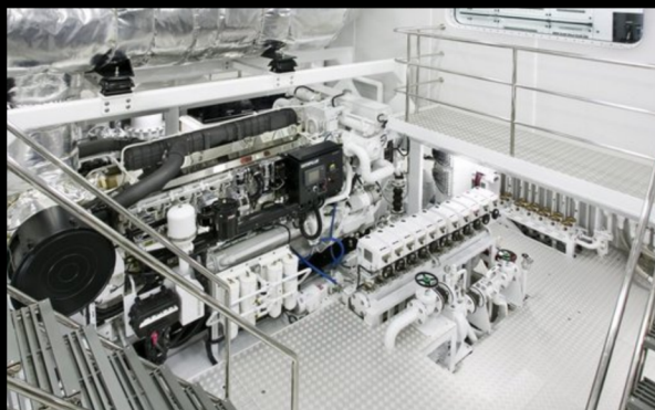
Engine Rooms & Cabins
