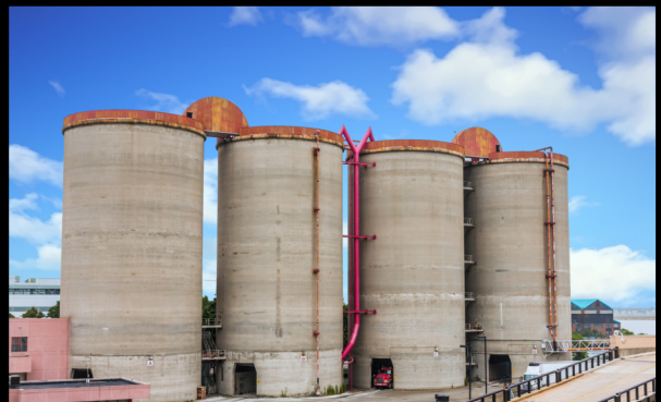
Grain Silos & Seed Storage Units
